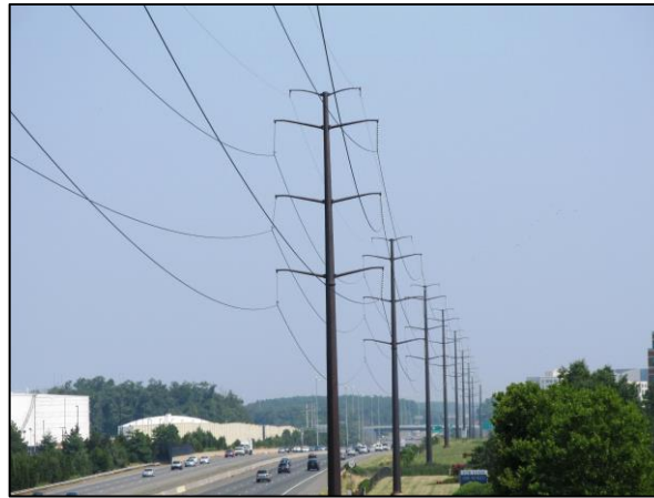
Examples of electric transmission double-circuit monopole structures. Not project specific.
