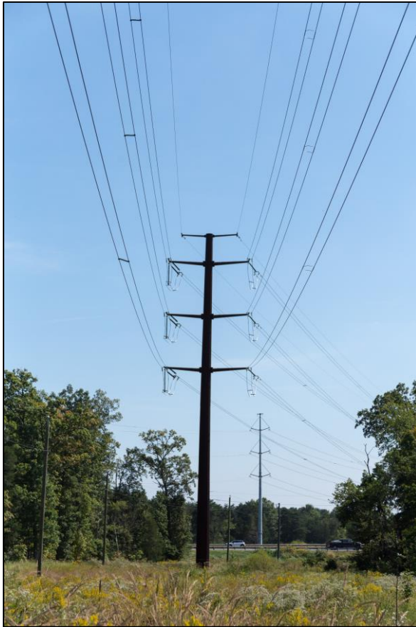
Examples of electric transmission double-circuit monopole structures. Not project specific.
