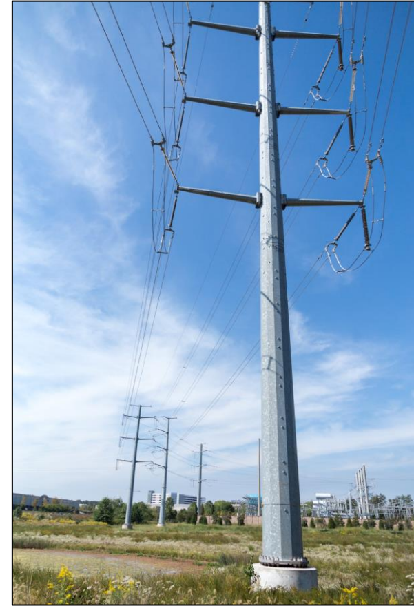
Examples of electric transmission double-circuit monopole structures. Not project specific.
